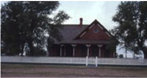
XIT GENERAL OFFICE BUILT IN 1898-99 TO HOUSE THE GENERAL OFFICES OF THE 3,000- ACRE XIT RANCH, THIS BUILDING SERVED THAT PURPOSE UNTIL THE FIVE- ROAD CARS OF BRICKS WERE BROUGHT IN TO CONSTRUCT THE OFFICE WHICH FEATURES VICTORIAN-ERA DETAILING IN ITS WRAPPING PORCH, DECORATIVE EAVE BRACKETS AND TURNED WOOD COLUMNS. DESIGNED TO IMPRESS VISITORS TO THE RANCH, THE BUILDING'S VICTORIAN FEATURES DISTINGUISHED IT FROM THE SURROUNDING RANCHING ENVIRONMENT. RICHARD TEXAS HISTORIC LANDMARK - 1754
